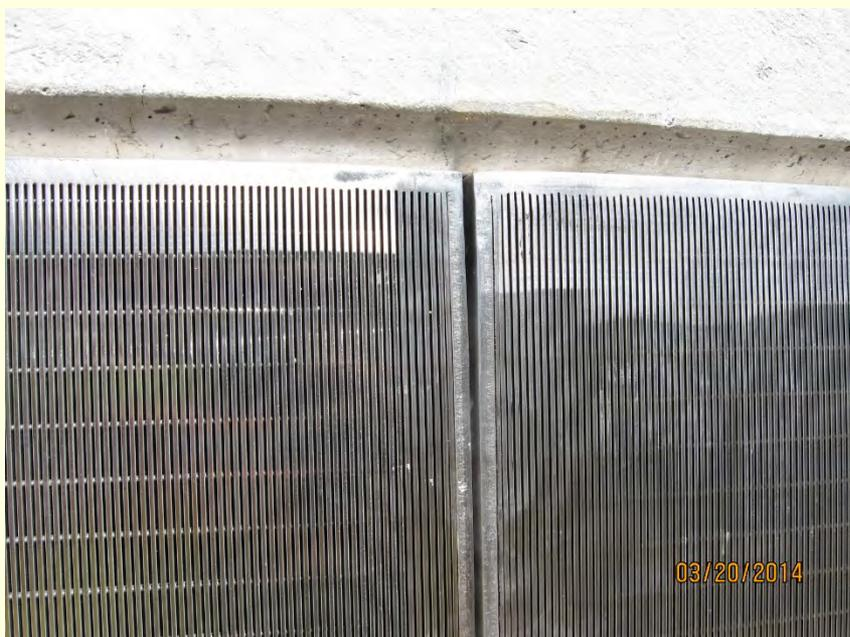
Fish screen panels constructed of V-wire profile bar with <math><0.0689</math>-inch width openings
